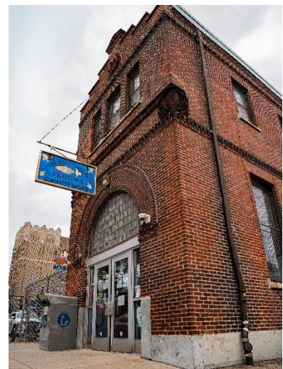
Fishtown Community Library has a new HVAC system, thanks to investment from the City's capital budget.
