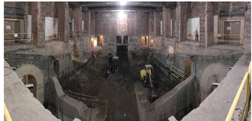
Space created within the heart of the Philadelphia Museum of Art by the demolition of the former Van Pelt Auditorium. A new public space called The Forum will be constructed here as part of the Core Project.
