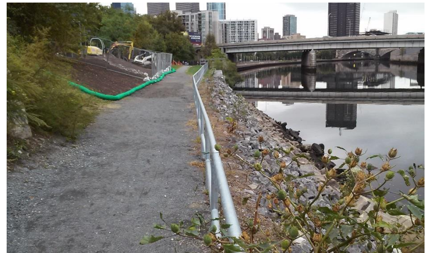
Reconstruction in 2017 of part of the Schuylkill River embankment and recreational path damaged by erosion in Center City
