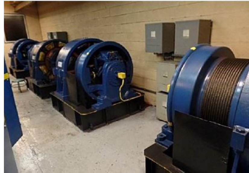
Existing Hi-Rise Elevator Machines, MSB
