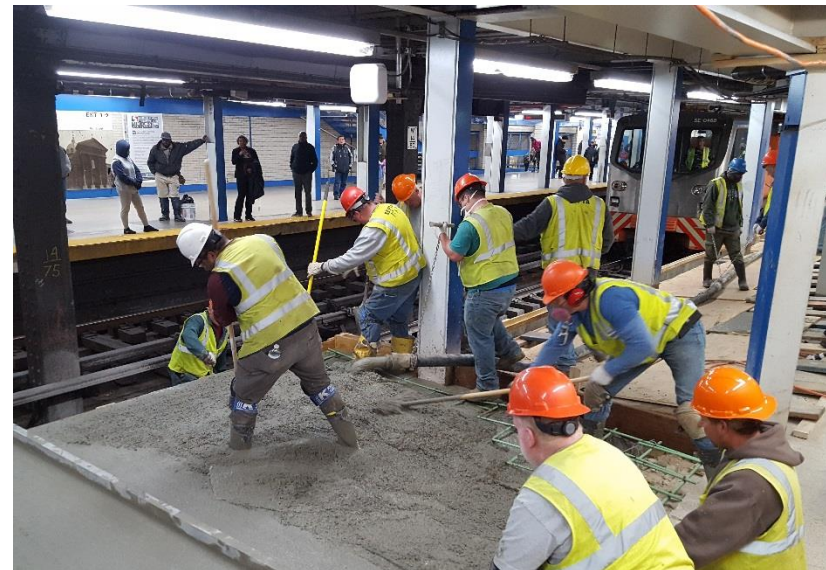
Market Frankford Line, Concrete Pour for Reconstructed Platforms, 15 th Street Station
