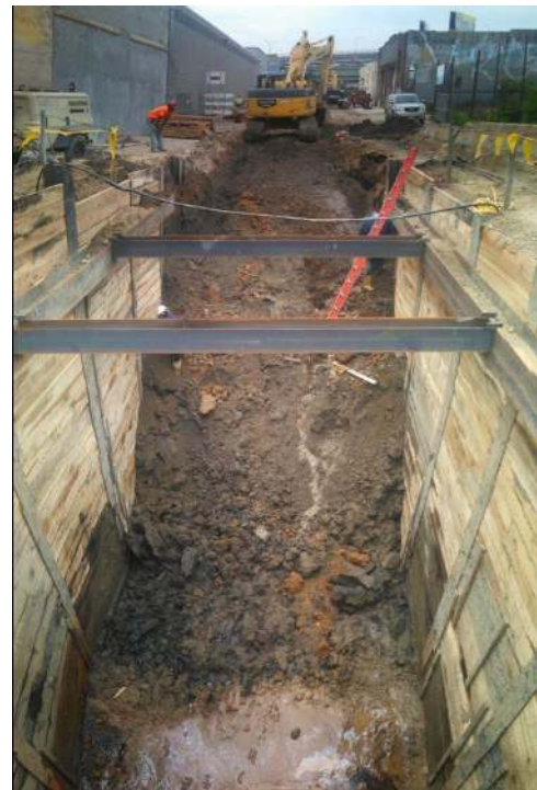
A large trench is excavated along Laurel Street for a box sewer, part of the Northern Liberties Storm Flood Relief project (NLSFR) to double the capacity of the system it is replacing.
