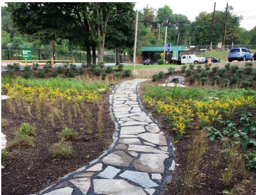
A thriving rain garden, constructed by the Philadelphia Water Department in 2016, drains over 38,000 sq. ft. of stormwater runoff in Germantown.
