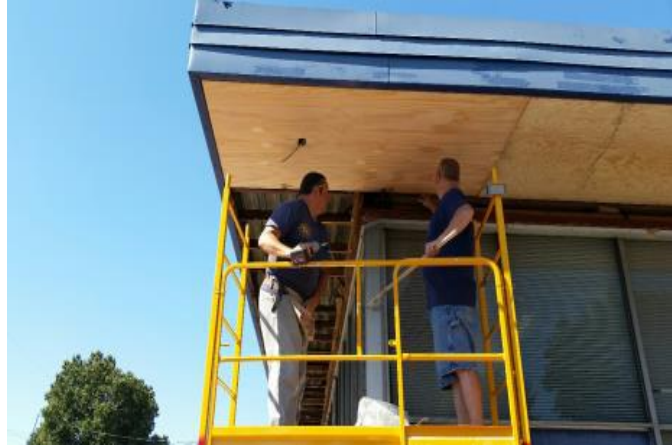
Police Tow Squad renovations in progress.
