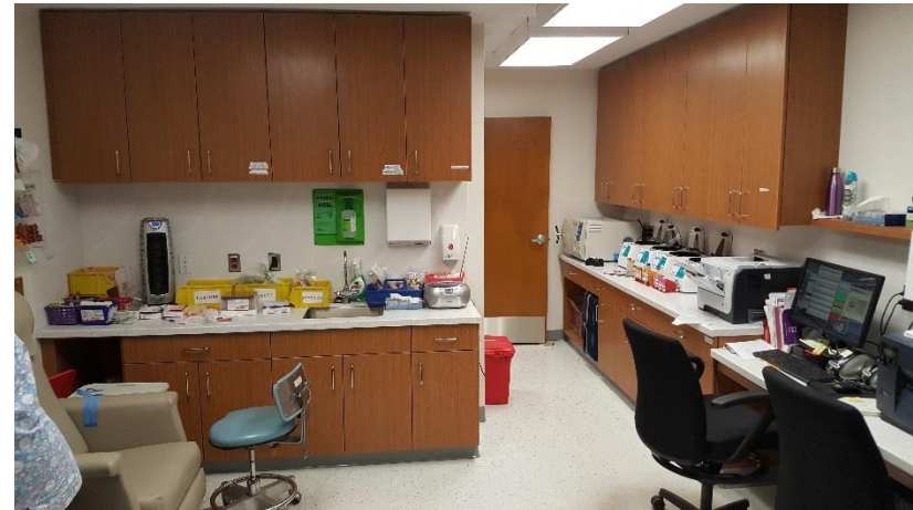
Newly renovated back office space at Health Center 10 on Cottman Avenue in Northeast Philadelphia
