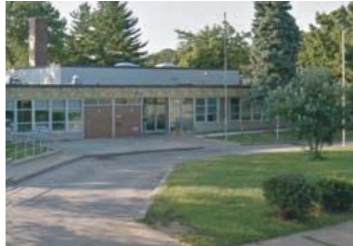
Stenton Family Manor, East Tulpehocken Street
