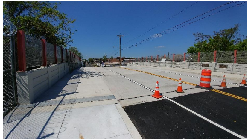
Reconstructed Sedgley Avenue Bridge over Conrail tracks in North Philadelphia
