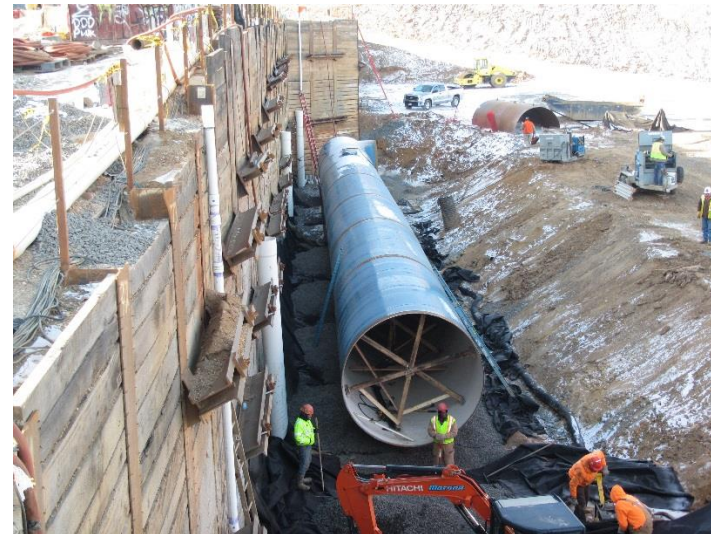
Philadelphia Water Department construction project in Northeast Philadelphia
