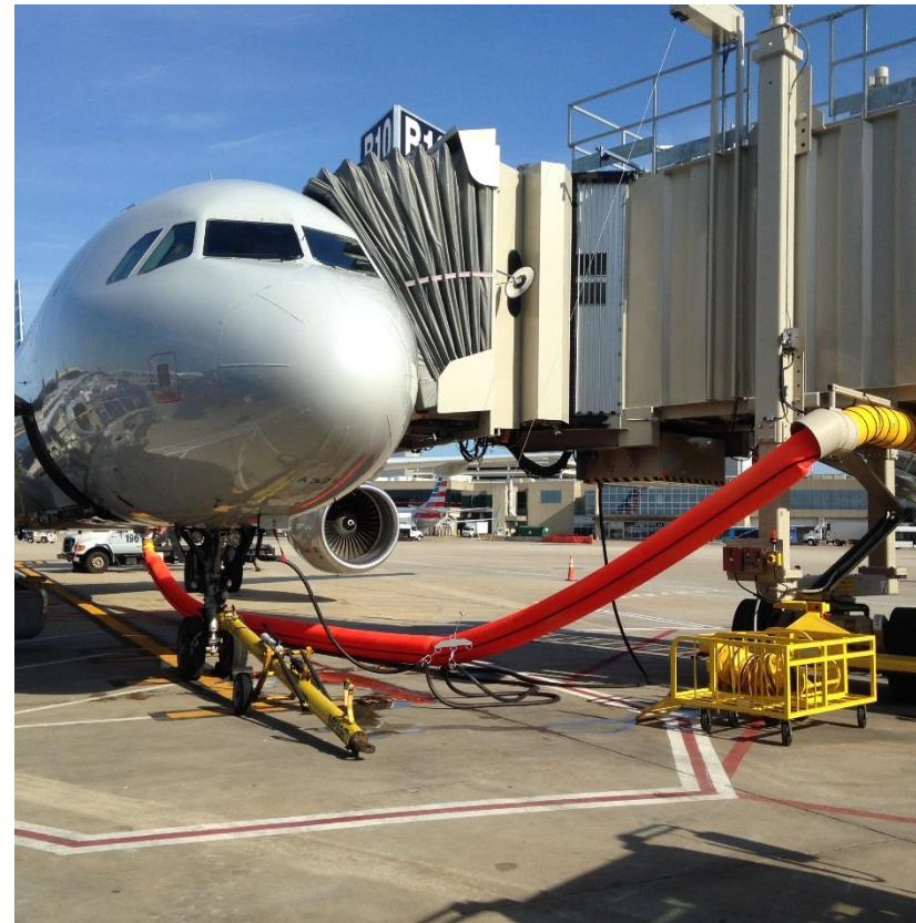
New passenger boarding bridge in operation at Philadelphia International Airport, Gate B10
