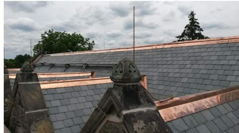
Recently restored roof at Engine 37, Chestnut Hill
