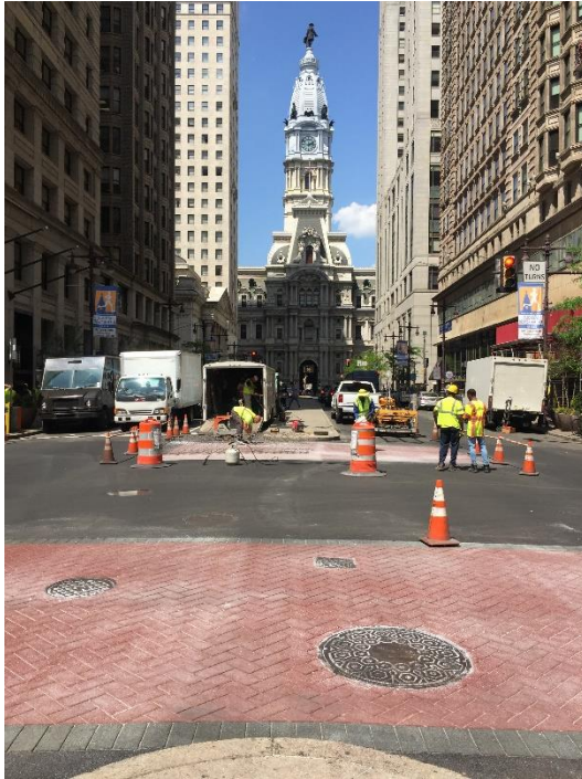
Streets installed a raised intersection on Broad Street.
