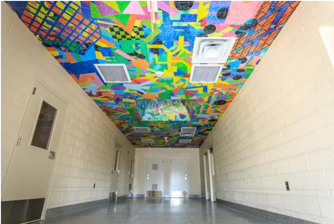
Art installed at Pleasant Playground in East Mount Airy as part of OACCE's Percent for Art Program.
